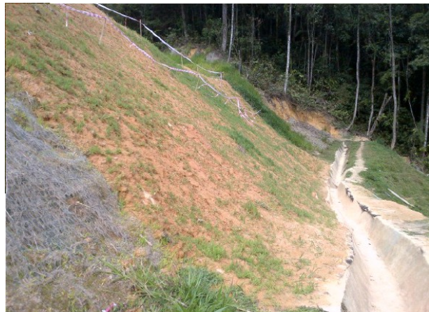
Plate 2: Slope protected with erosion control mat and drainage net, managed to prevented failures.
